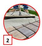
Sweep with a push broom in all directions so joints are filled.
