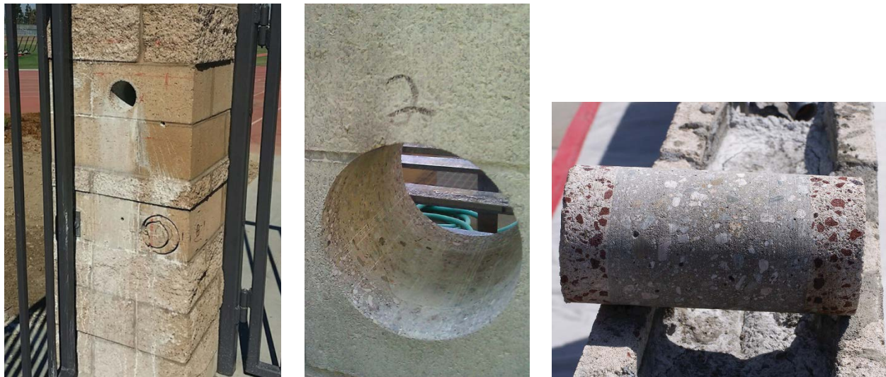
Figure 3. Illustration of the Destructive Nature of Coring
