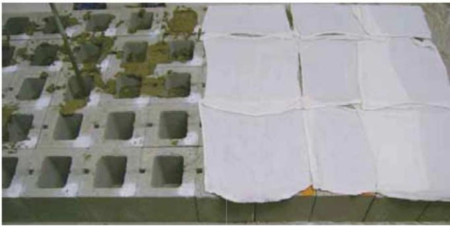
Figure 2: Grout samples during casting.
