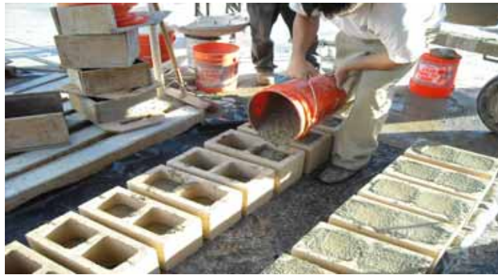
Figure 1: Grout Placement in Concrete Masonry Unit Cells
