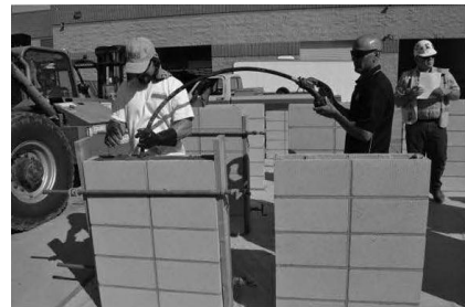
Figure 5: Consolidating Grout
