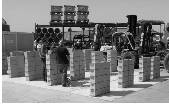
Figure 3: Masonry panels prior to grouting (bond beams mortared to restrict grout)
