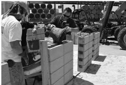
Figure 4: Bucketing Grout into Sample Panel
