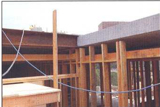
Second floor spancrete diaphragm.
