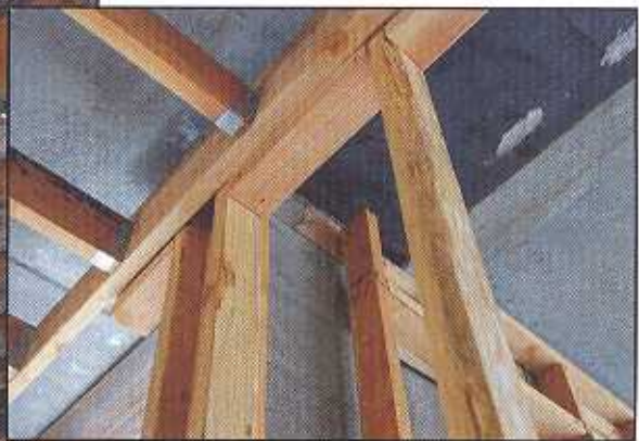
Interior non-structural wall connections.
