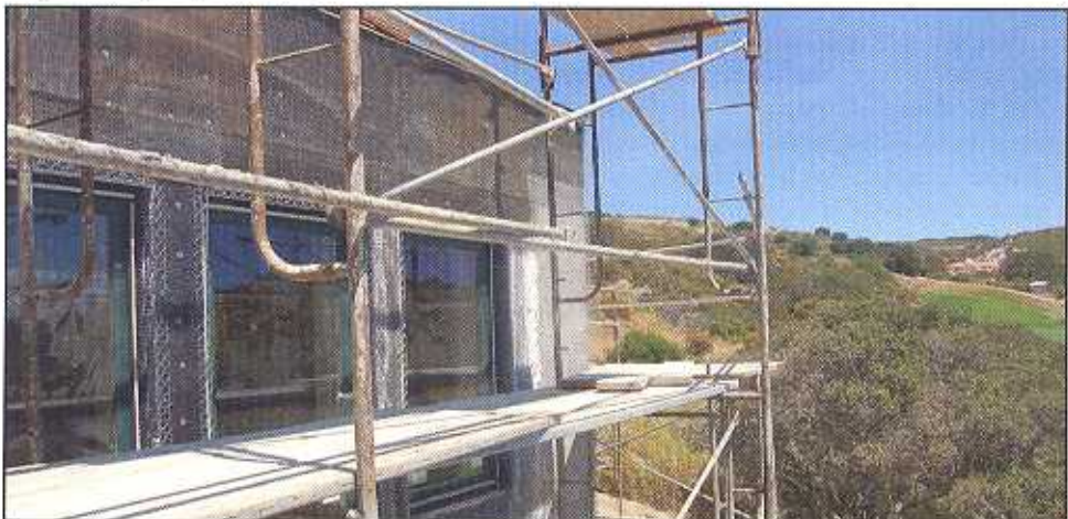
Exterior masonry application.
