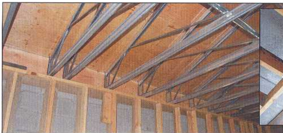
Roof Truss Diaphragm connection.
